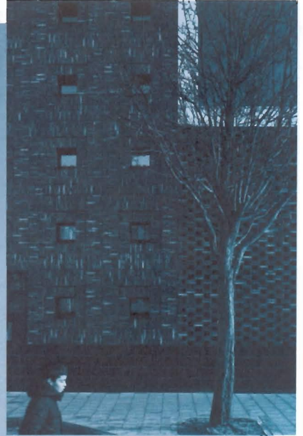
Fig. 55 - detail of masonry
